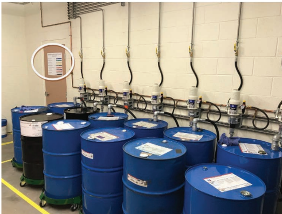
Figure 1: These bulk storage containers have color-coded magnetic strips on the top of each to match the chart on the door to the far left.
