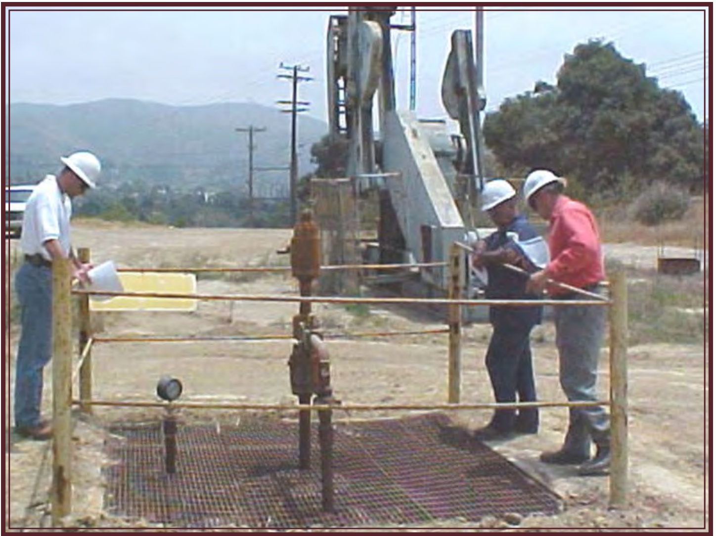
Vice-President of Operations (l) and Manager of Operations (r) inspecting equipment as part of a Leadership Audit in Ventura
